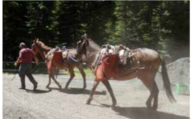
Mules, each carrying 200 pounds of gravel 1.2 miles one way to bridge and trail repair. Several trips were done for this trail and bridge repair. And it was hot, hot, hot.
