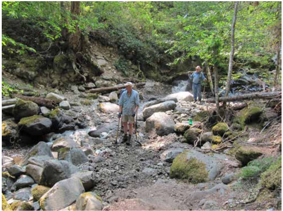
Boulders that caused leg trap were removed from the creek. Marty DeVall and Jerry Bentz gathering tools after finishing Work Area 3.
