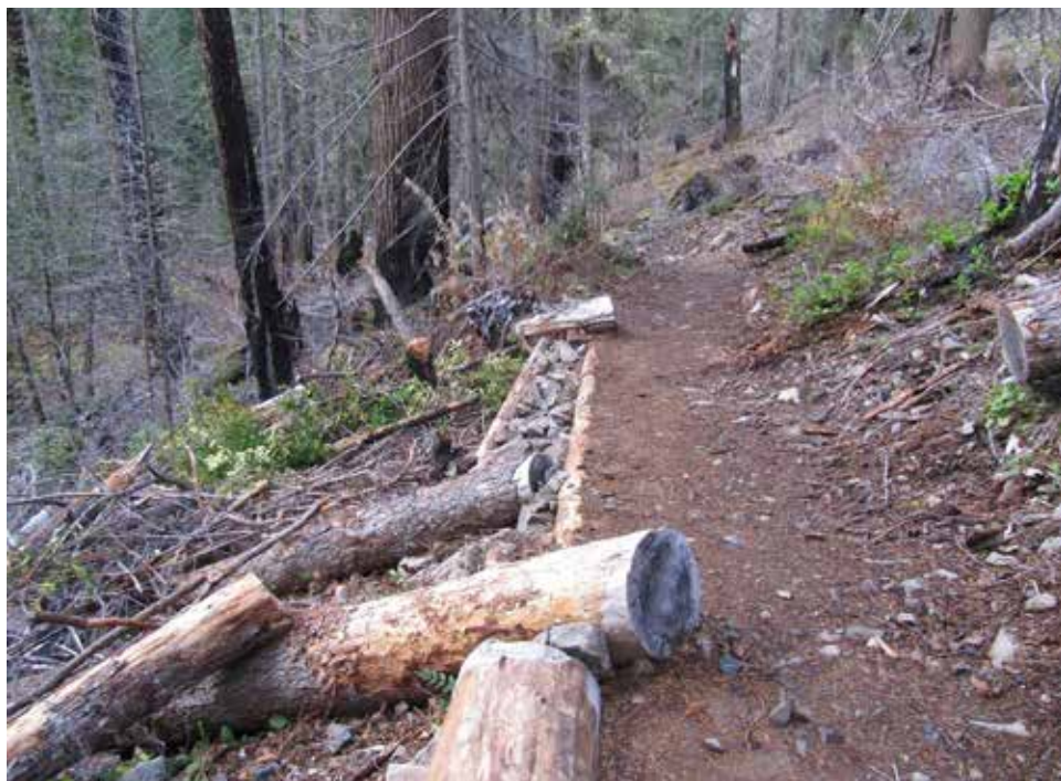
Northwest Youth Corp built numerous log cribs and back-filled the trail to cover and restore the rocky, burned areas in Work Area 1
