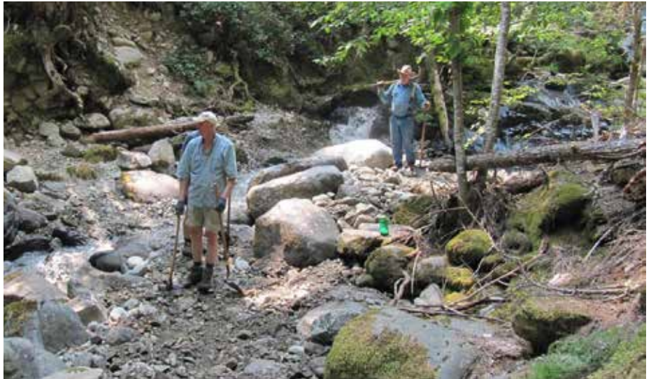
Boulders that caused leg trap were removed from the creek. Marty DeVall and Jerry Bentz gathering tools after finishing Work Area 3.
