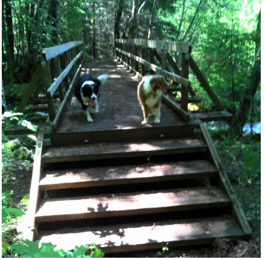
Figure #5: N43 degrees 29' 45. 77" by W122 degrees 23' 58.61", Middle Fork Willamette Trail. Large bridge with steps. Bridge in good shape, but the approach is stair steps, which are potentially dangerous to horses and riders. These need to be replaced by a ramp.
