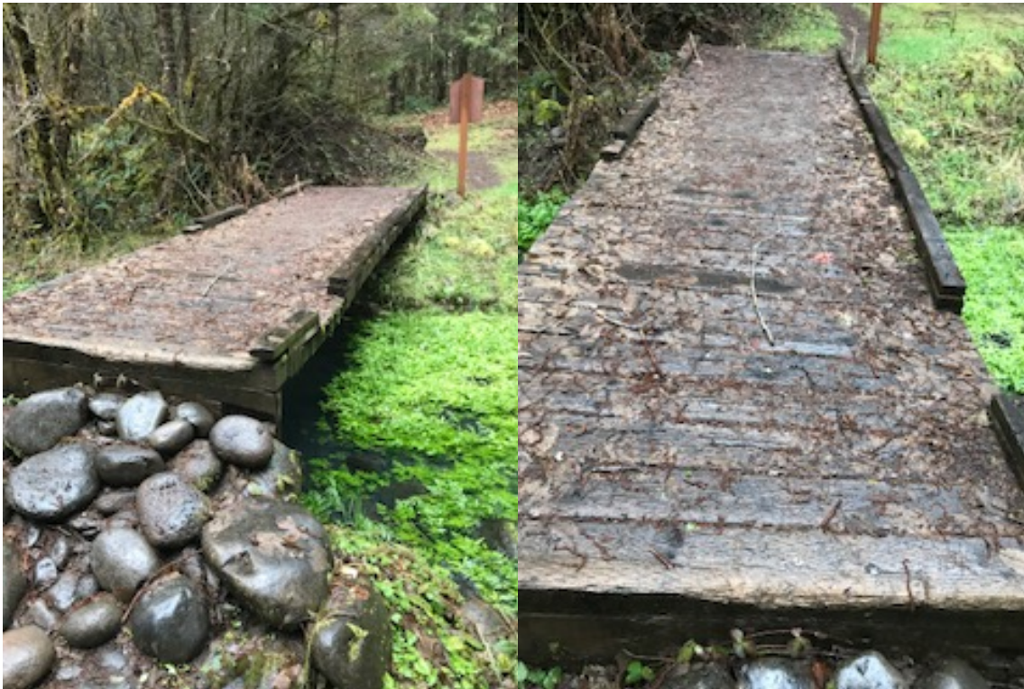
FIGURE #2: N43 degrees 34'527" by W122 degrees 27'694", Middle Fork Willamette Trail. Bridge too slippery, too narrow and not weight bearing for horses. Horses cannot use this improvised bicycle bridge and so are forced to drop down approximately 2 feet off muddy bank into slough where they sink into mud and heave themselves up onto opposite bank.
