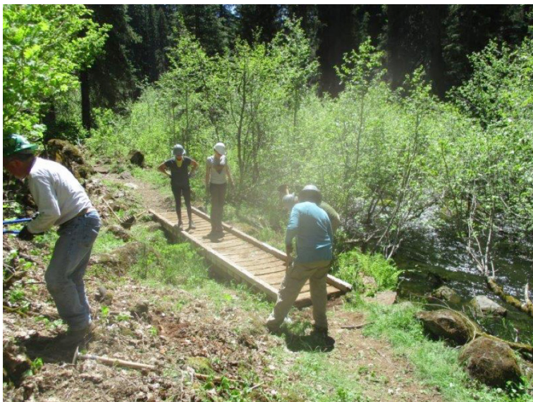
PCTA crew brushed out Puncheon that was overgrown with brush.
