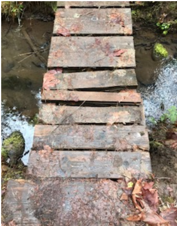
FIGURE #2: N43 degrees 34'527" by W122 degrees 27'694", Middle Fork Willamette Trail. Bridge too slippery, too narrow and not weight bearing for horses. Horses cannot use this improvised bicycle bridge and so are forced to drop down approximately 2 feet off muddy bank into slough where they sink into mud and heave themselves up onto opposite bank.
