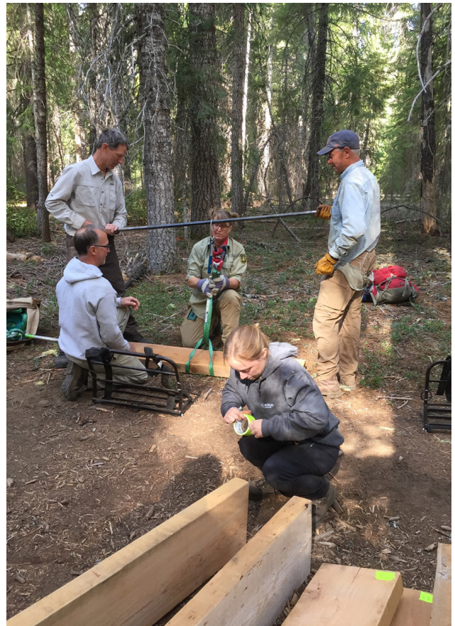
Upper Rogue River USFS Crew at work assisting the Sourdough Chapter pack in of bridge timbers and equipment Aug 31 – Sept 3, 2020
