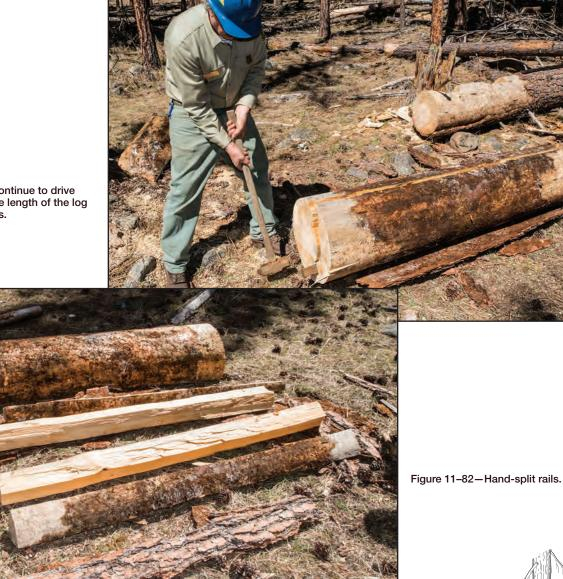
Figure 11-81 - Continue to drive wedges down the length of the log until the log splits.
