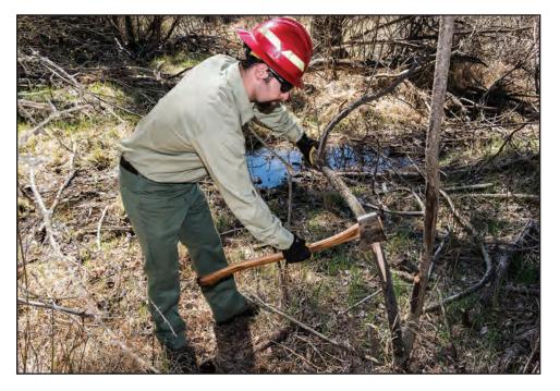
Figure 11-28-Using a one-handed swing to cut a small sapling.
