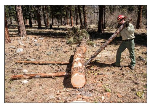
Figure 11-64-Using a lever to move a log.
