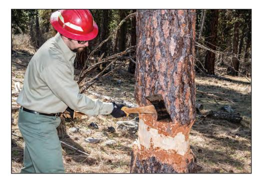
Figure 11–49—Clearing bark from an area on a tree before using a crosscut saw.
