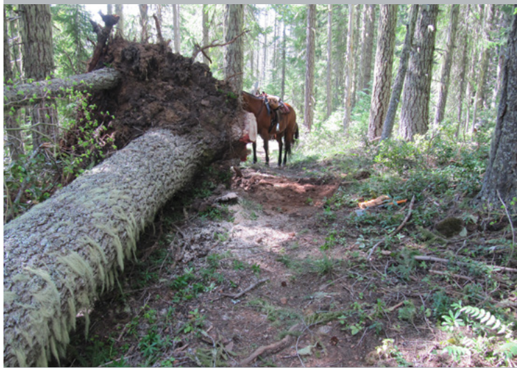
Finally the dirt was cleaned off the roots to allow us to cut away a large section. This allows rider and pack animals to easily clear the area around the tree rootwad. Dirt was also replaced in the trail to fill the holes caused by the root upheaval.
