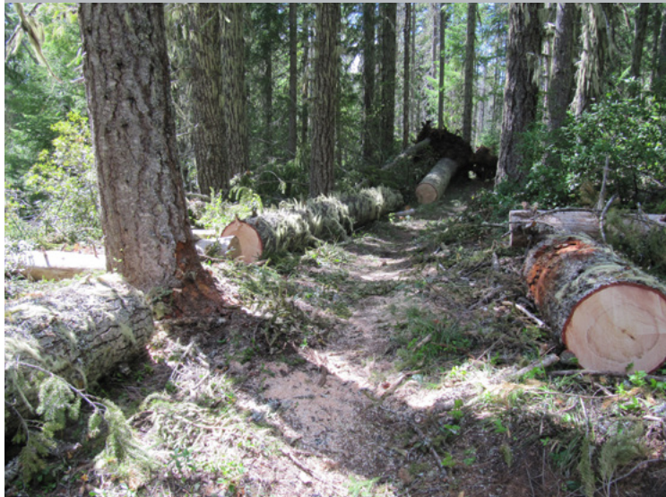
Logs from the upper portion of the tree were cut away. Smaller logs were placed under about a 30 foot section of tree. The section was cut, which came down on the logs allowing us to easily roll it off the trail.
