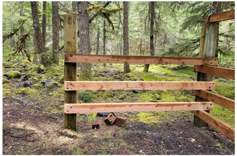
Site 9 post repair
