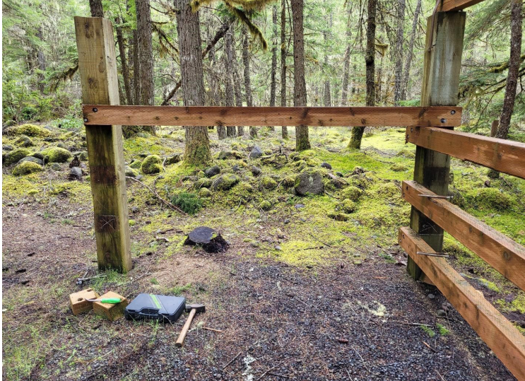
Site 9 Corral with two missing rails. Just the end pieces were left and were removed prior to the photo taken
