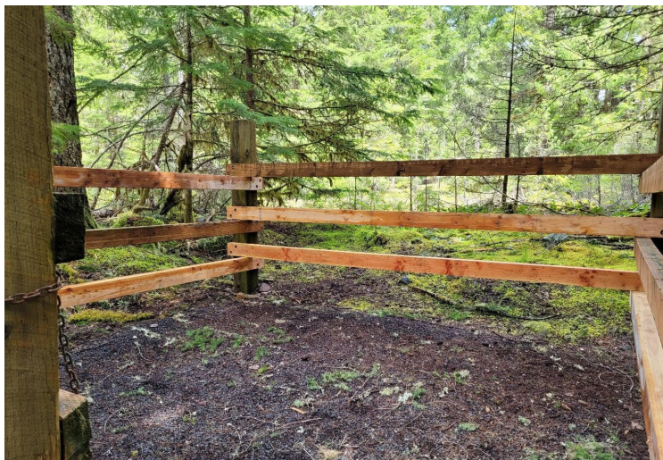
Figure 3. Repaired using 4 in x 6 in x 14 ft rails.
